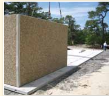
Easi-Span Building being assembled.
