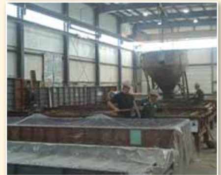
Barrier forms being poured at CJ Pink.
