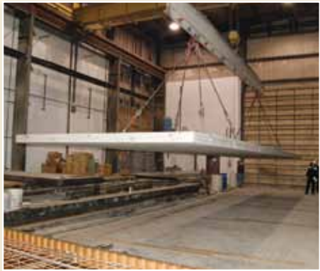
Prestressed floor panel in production.
